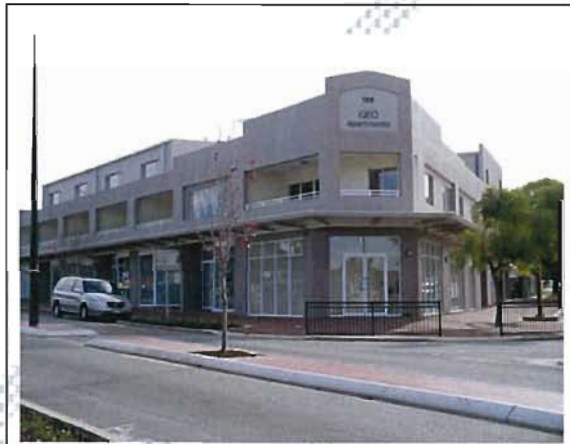
This 3 storey mixed use development combines ground floor retail/commercial uses with residences above. The third floor is set back from the street alignment, thereby reducing the apparent overall height of the building in the streetscape.
