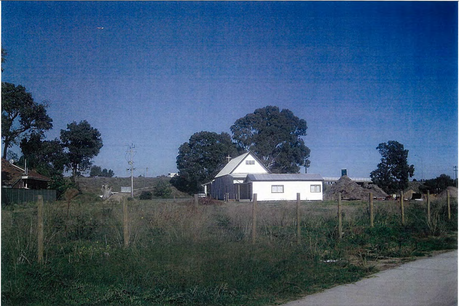
Additional Place of Worship Building Lot 387 (506) Welshpool Road East, Wattle Grove Photograph of the Property from Sessilis Crescent
