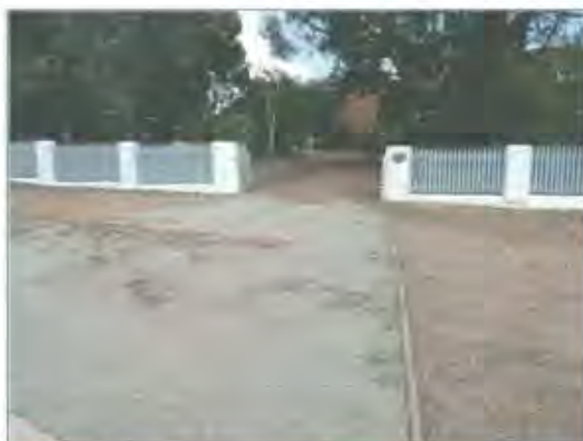
Photo 3: Existing Site Access
