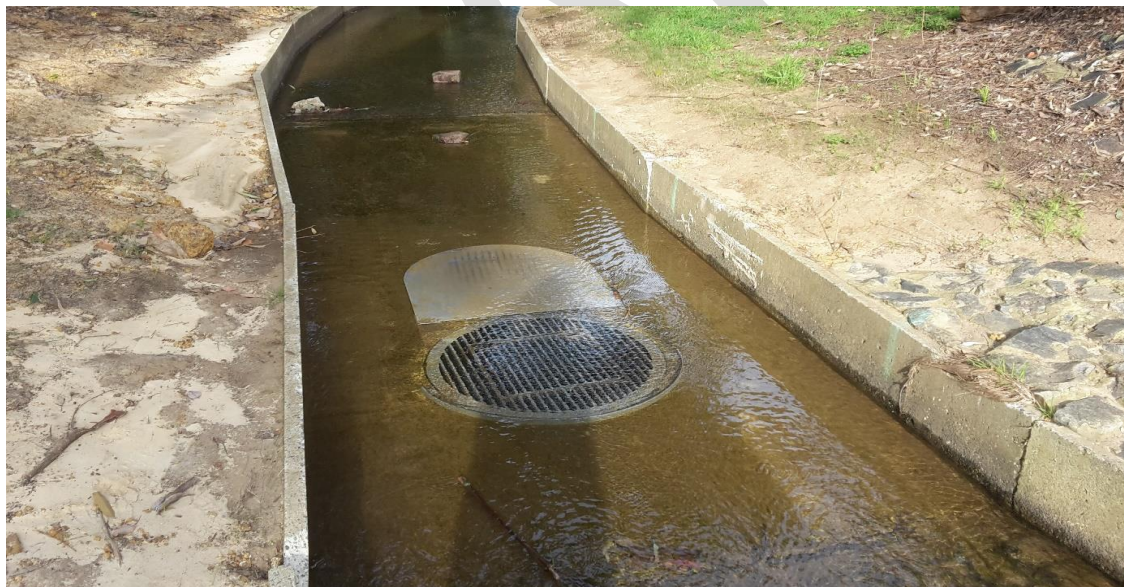
Woodlupine Main Drain stormwater extraction point
