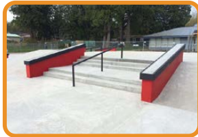
4. STAIRS, LEDGE & HANDRAIL
