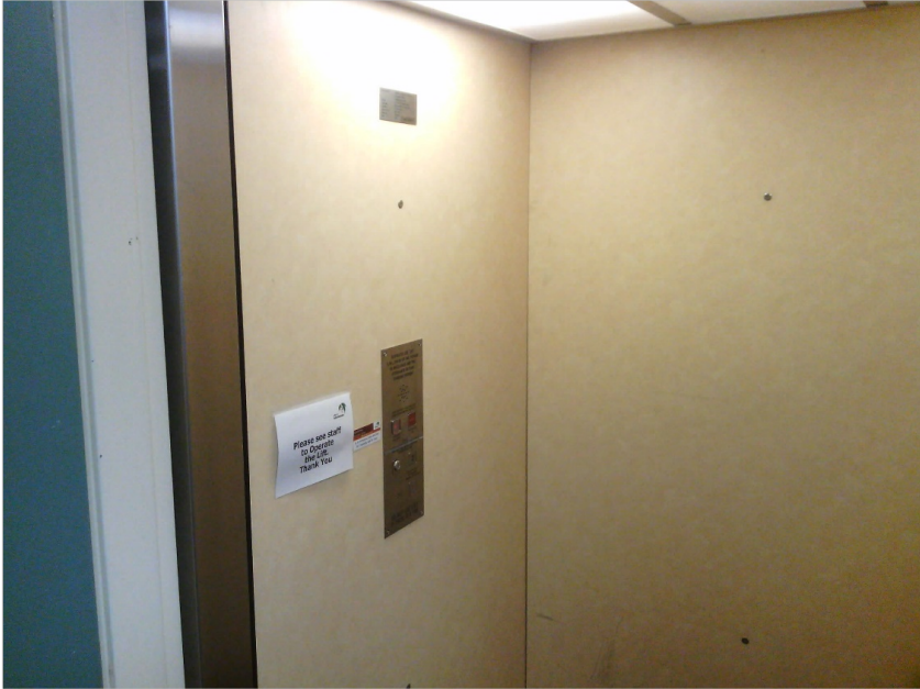
Repair of lift
