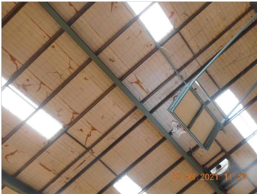
Replacement of roof sheeting and lining
