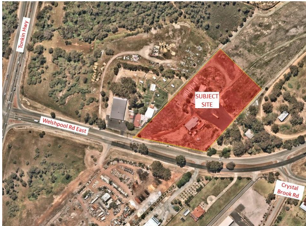
Figure 1: Aerial view of the subject site (currently under construction)
