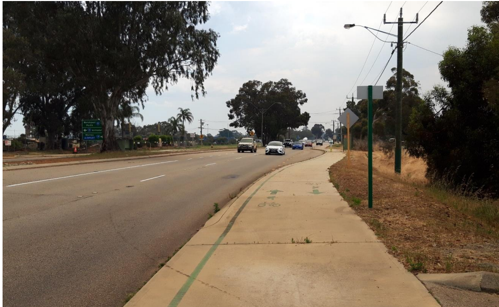
Figure 4: Westbound view along Welshpool Road East in the vicinity of the future garden centre crossover
