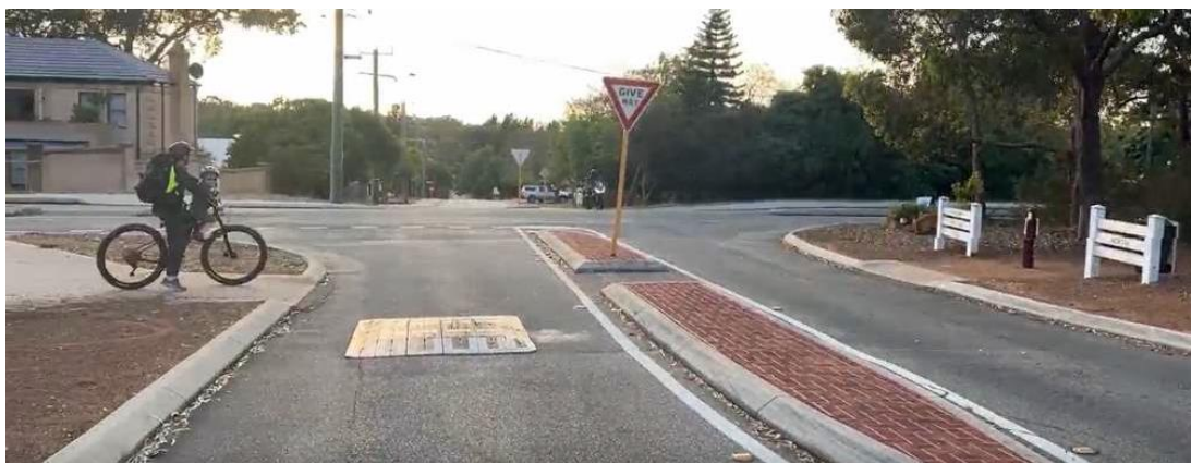
Photo 10: Mid-block Pedestrian crossing on Elizabeth St
