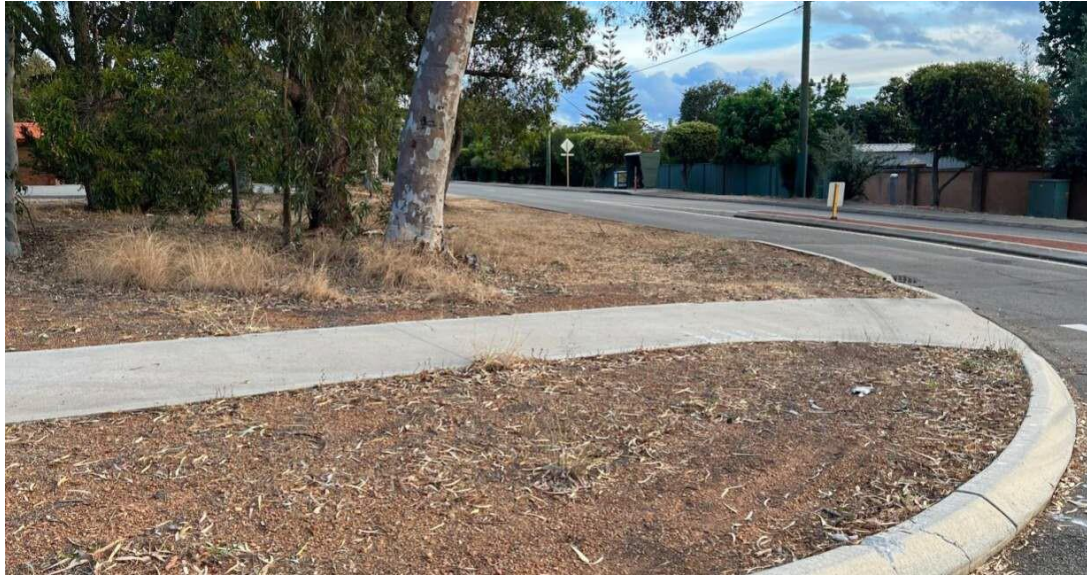
Photo 4: Sight Distance is also limited to the South on Elizabeth St Westbound
