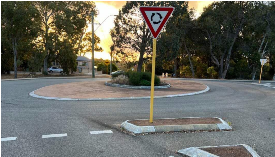
Photo 6: View from Eastern Leg of Roundabout Towards the Western Leg
