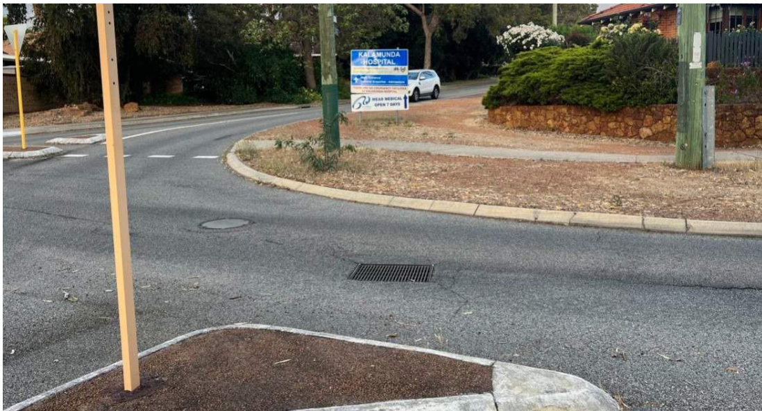
Photo 8: View Towards the Eastern Leg that is Partially Obscured by Kalamunda Hospital Sign
