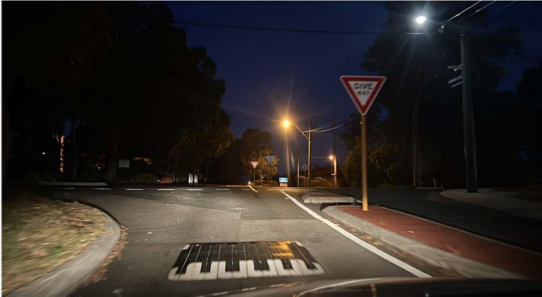
Photo 12a: Dim Lighting of Elizabeth St/Railway Rd intersection, view westbound
