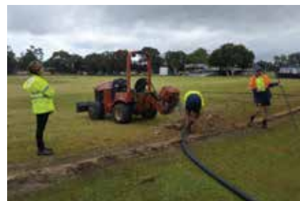
Scott Reserve cricket ground irrigation replacement at minimum inconvenience to the grounds use.
