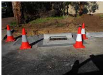
New side entry and kerb replacement
