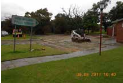
Public car park Box out of old surface
