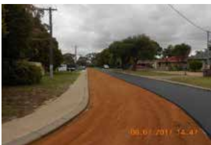
Profiled area with section with 25mm SMA base layer
