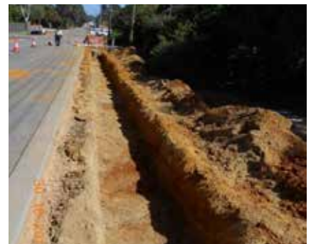
Drainage works in progress
