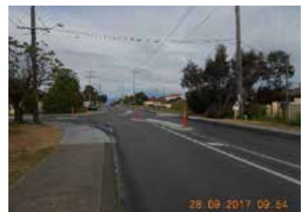
Completed civil works
