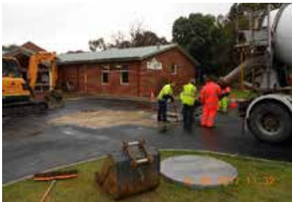
New storm water grate
