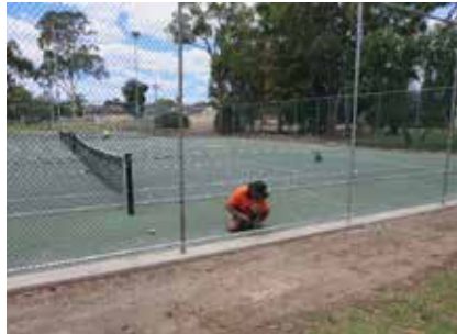
Fencing and Flush Kerbing during
