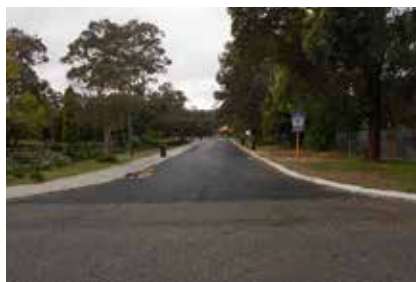
New path install
