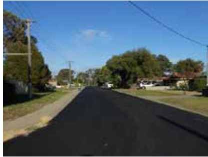
Completed works with 25mm dense grade wear layer
