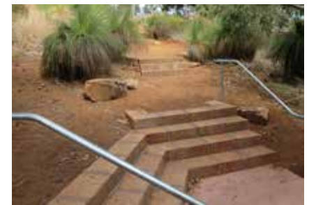
New Stairs from top of Nangana New Steps and Handrailing at bottom of Nangana
