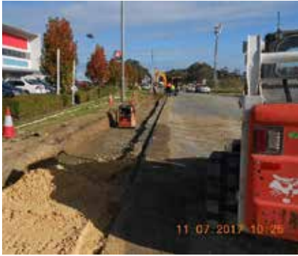
Completed works with 25mm dense grade wear layer
