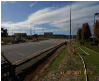
Civil works consist of boxing out for widening and installing new base coarse
