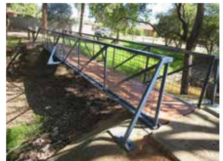
Re-decking and painting of the existing bridge
