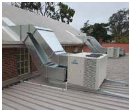
New Air conditioner units to the Kalamunda Agricultural Hall
