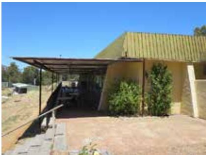
Main Verandah Area - Before
