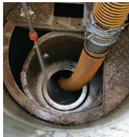
Hartfield MAR extraction well.
