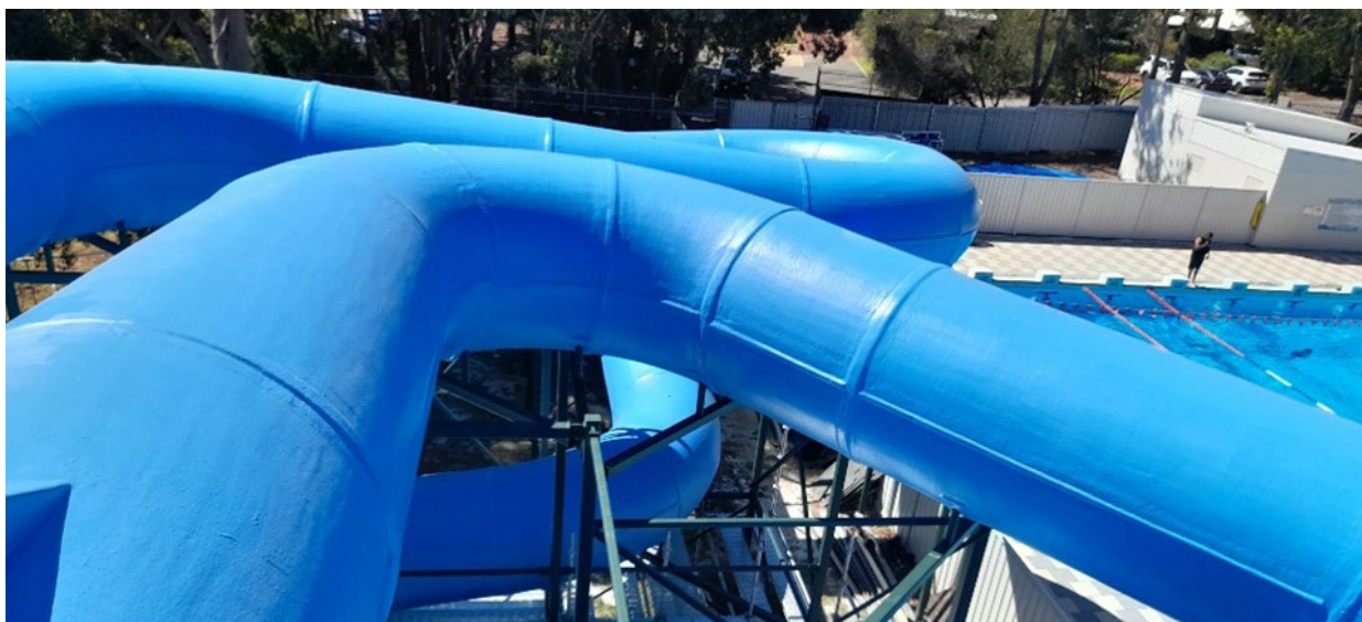
Pictured: KWP New Gelcoat Applied
