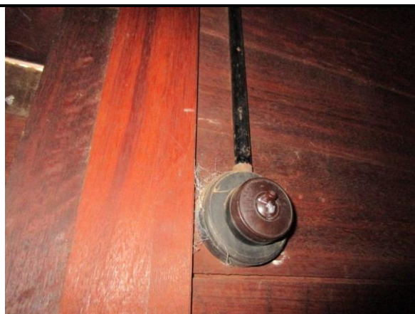
Photos from March 2021 inspection.
