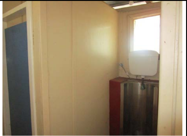
Photos from March 2021 inspection.
