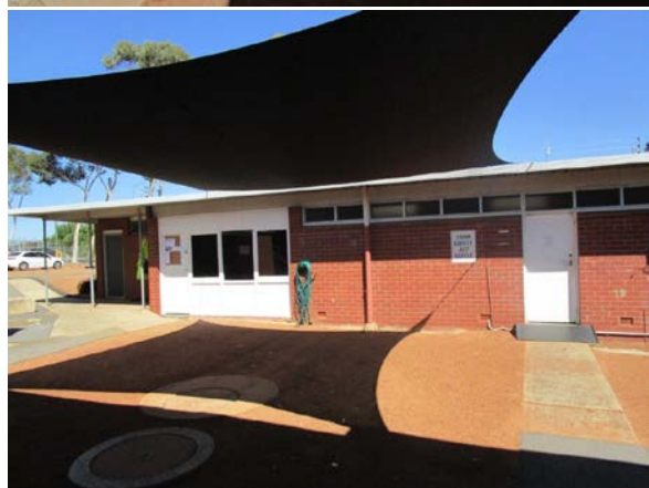
Photos from March 2021 inspection.
