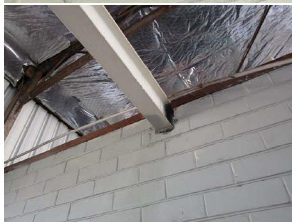
Photos from March 2021 inspection.
