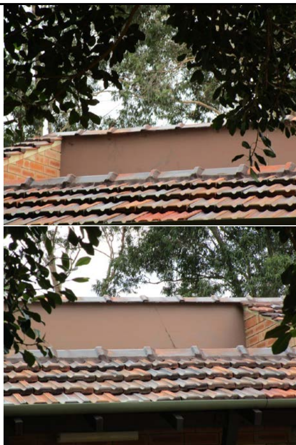
Photos from April 2021 inspection.
