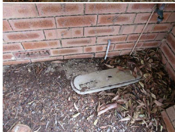
Photos from April 2021 inspection.
