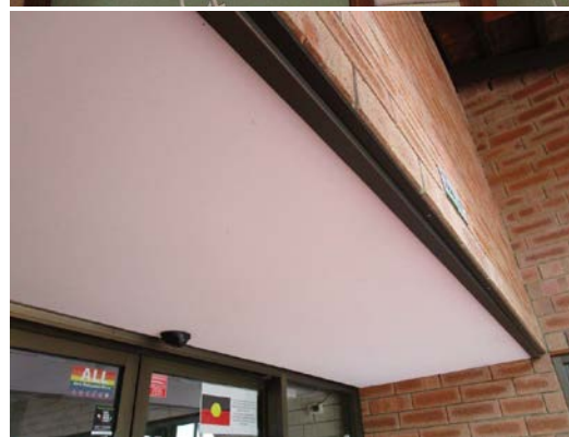
Photos from April 2021 inspection.
