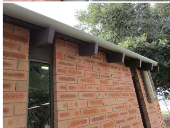
Photos from April 2021 inspection.
