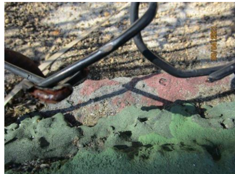
Photos from April 2021 inspection.
