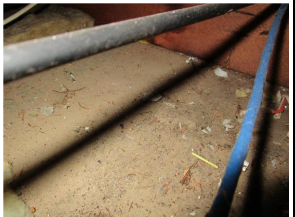
Photos from April 2021 inspection.
