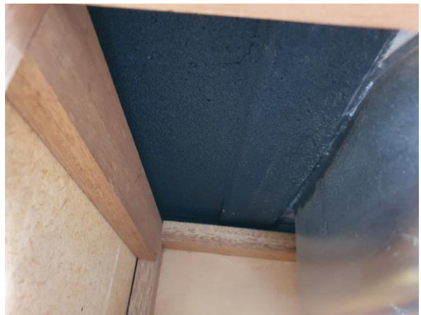
Photos from April 2021 inspection.
